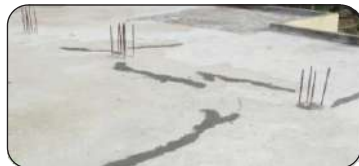
Fill Chemical in Cracks
