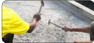
Removing Loose Material
