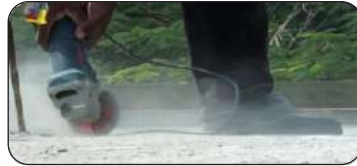
Opening Cracks in V Groove Shape
