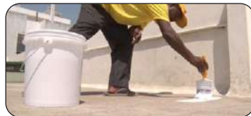
1st Coat Penetrative Heatproofing
