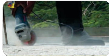
Opening Cracks In V Groove Shape
