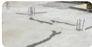
Fill Chemical In Cracks
