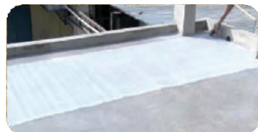
Laying Fibremesh
