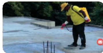
1st Coat Penetrative Waterproofing
